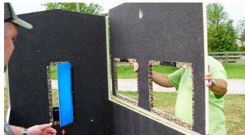
Starting with the right back upper horizontal panel with vent, insert pre-caulked panel into back panel and on top of bottom panel. *Note: Make sure vents are located on opposite walls-one on the upper panel and one on the lower panel.*
