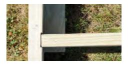
Align remaining cross brace joists **(#3)** in dado slots and attach with 2 screws per attachment point.
