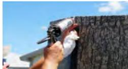
Vertical seams on the roof hem. *Hint: apply caulk and then wipe from bottom to top to be sure to seal the upper edge of the vertical seam opening.* Roof extrusion cover cap-caulk the vertical seams of the cover cap.
