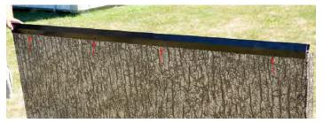
Using (4) of the 3/4" pan head screws, attach the extrusion to the roof panel in the following order: Place one screw 5" in from each end of the extrusion. Add the remaining two evenly between each end screw. Repeat procedure for the 2nd roof panel.
