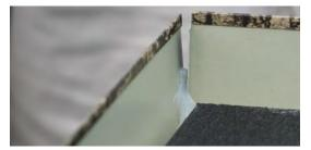
Caulk all roof interior vertical seams with clear caulk from the bottom to half way up the opening (do not smooth out with finger). The goal is to seal the opening near the SIP panel but leave the ends open so they can flex when installing the roof.
