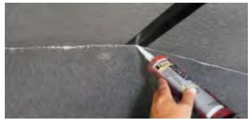
Run a bead of black caulk around the upper interior perimeter where the roof meets the walls. Smooth with finger to seal the seam. Allow the caulk to dry based upon manufacturer's recommendation on tube.
