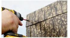
Lift the roof over the blind and gently lower onto the blind walls. Starting at the left back panel and working 1/2" up from the bottom edge of the roof, use 3/4" pan head screws to attach roof to each corner in a clockwise fashion.
