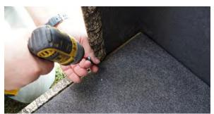
Attach with (3) screws per side ensuring to catch the floor frame below the OSB for a secure fit. Hint: Angle the screws at the Door panel 45 degrees.
