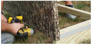
Starting with the back panel, center the panel on the end joist and hold in place. Working 3/4" up from the bottom edge add screws every 4"-5" to secure back panel in place.
