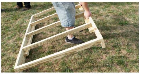
Flip the floor back to the upright position and check for square one last time.
