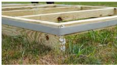
Working 1/2" down from the top edge of the board, attach the adhesive tape around the perimeter of the rectangle. Do not overlap the tape at the start and end points.
