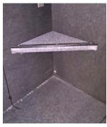
Place shelf along the back left corner so the bottom edge is approximately 14.5" above the floor. Note: the floating bracket should be placed against the left side panel.
