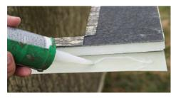
Add clear caulk to the upper horizontal side panels (metal overhang portion) by running a zig zag bead from end to end.
